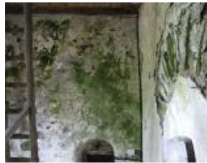
Damp on the tower room walls before the work.
