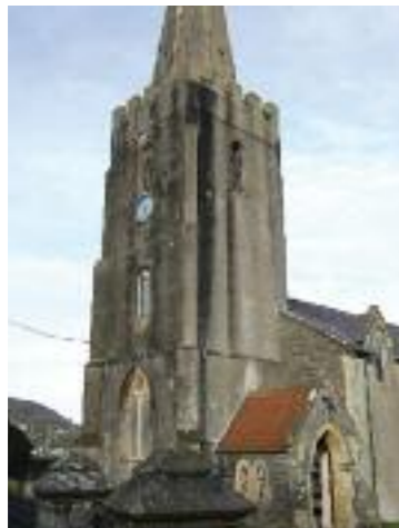
St Patrick's Church tower before renovations.
